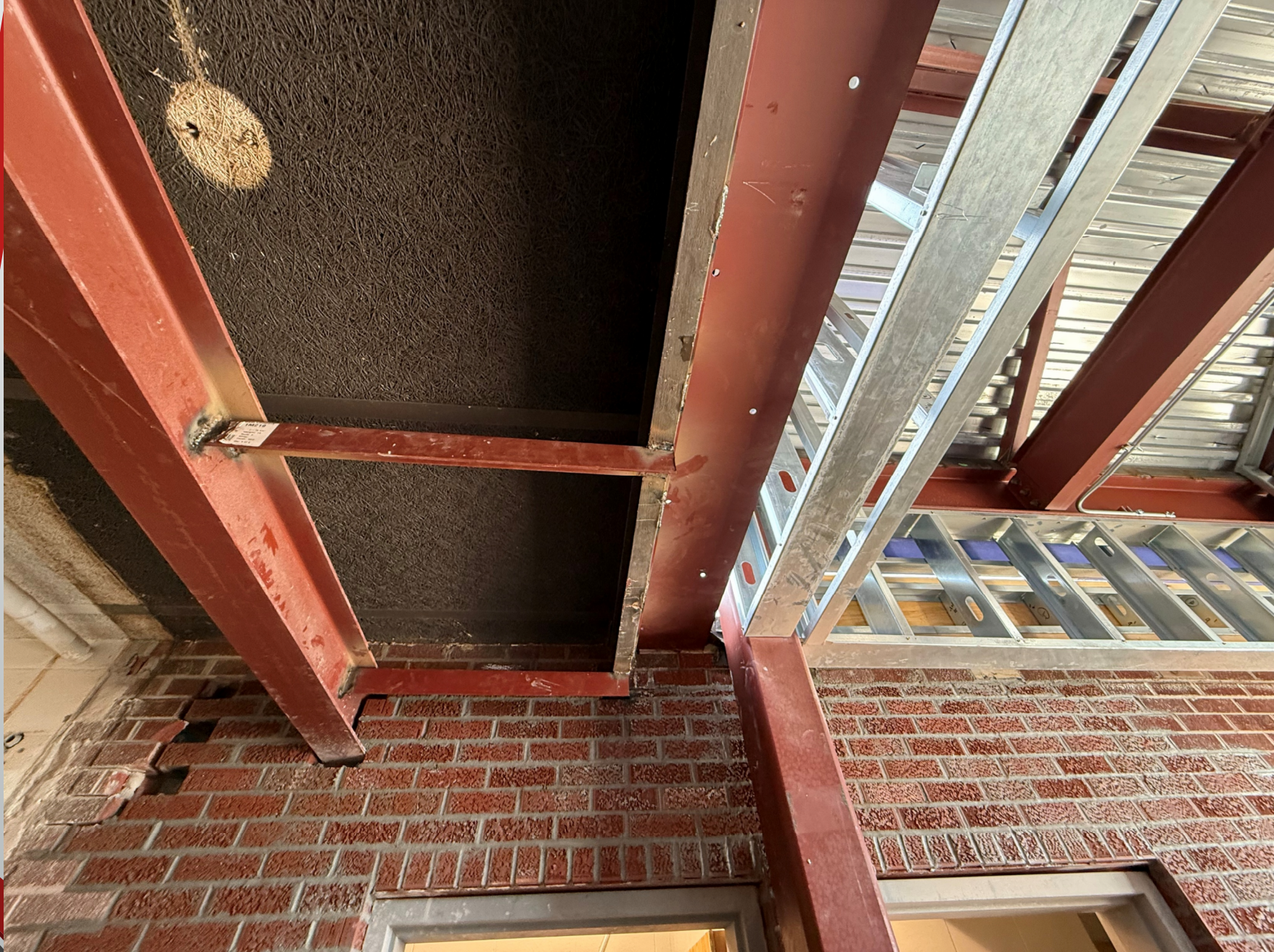
Installed additional structural steel at new High School Entrance to tie in the two different roofs
