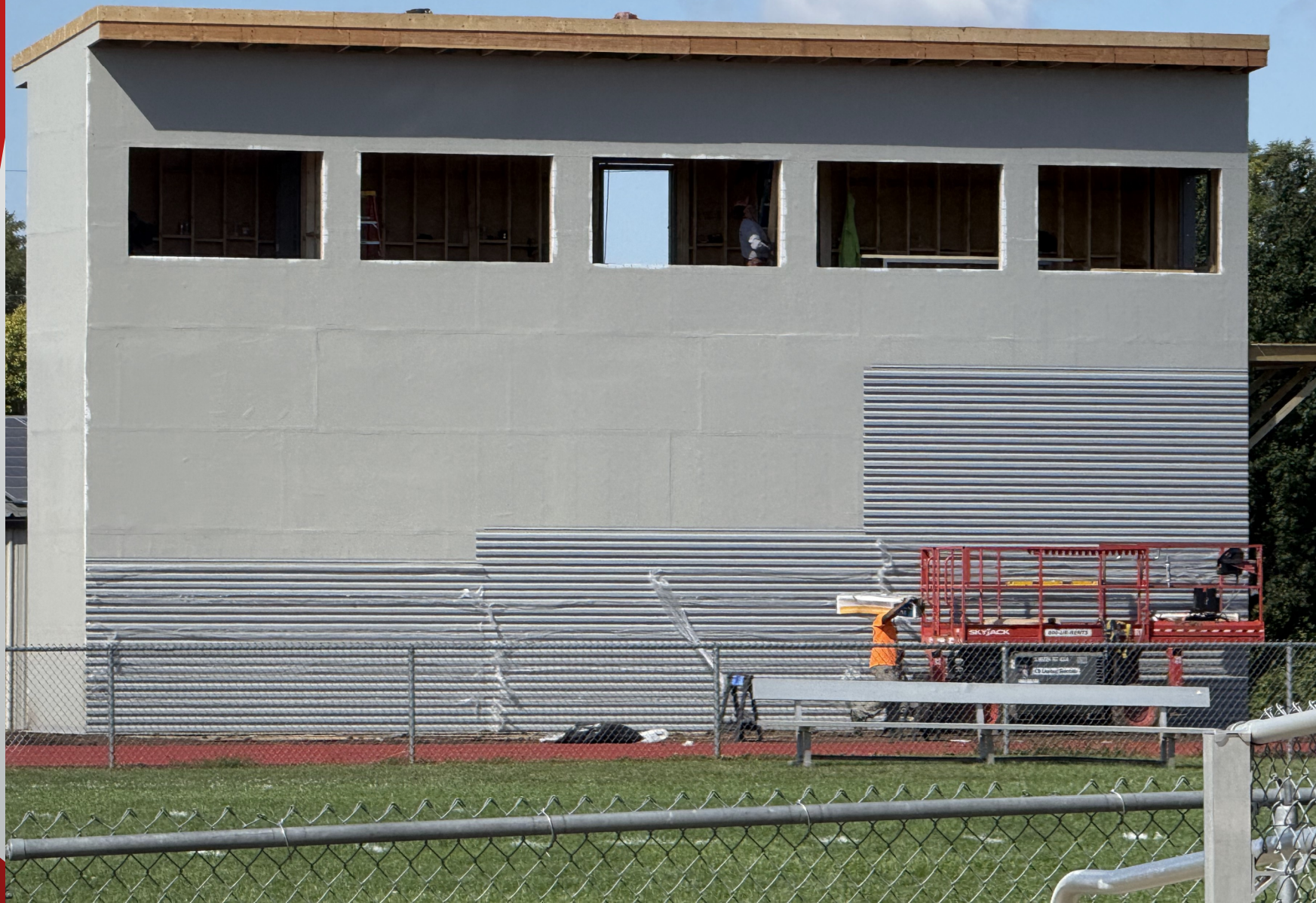
High School press box framing completed and started on installing metal wall panels
